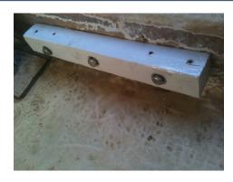
I then used lag bolts to attached the 2x4s to the 1.5 inch mounts. This allowed the 2x4s to be even with the string height. Finally, the drip pan was installed on top as a final support.
